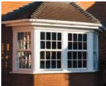
Bay window with vertical sliding sash windows
